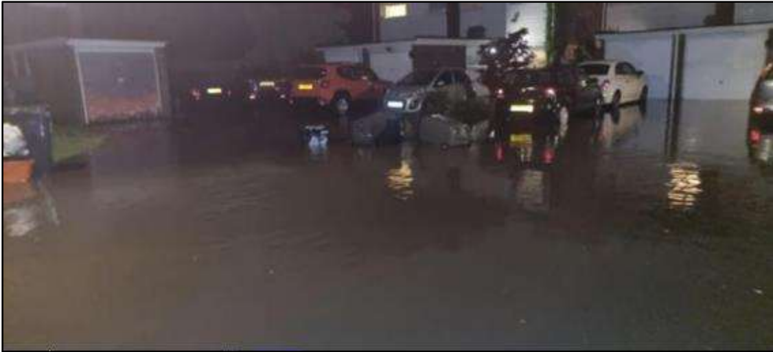
Figure 9 Photo showing flooding to residential carpark area
