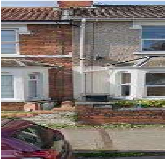
Figure 20 Shared roof drainage downpipe discharging onto the highway footpath in Montagu Street
